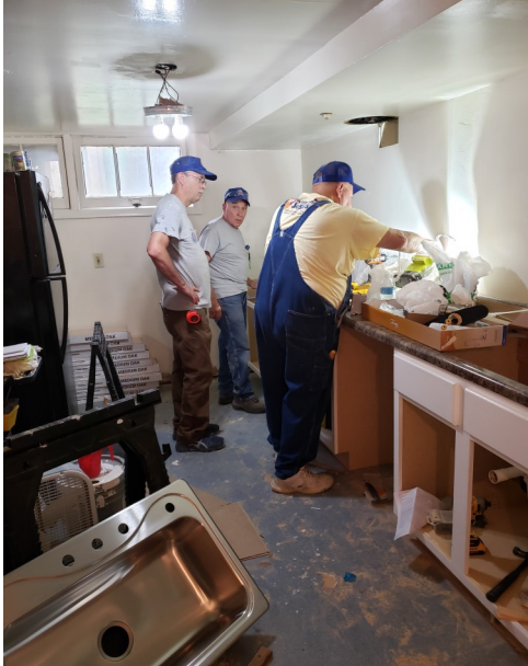
July —remodeling the basement apartment for IBSA.
