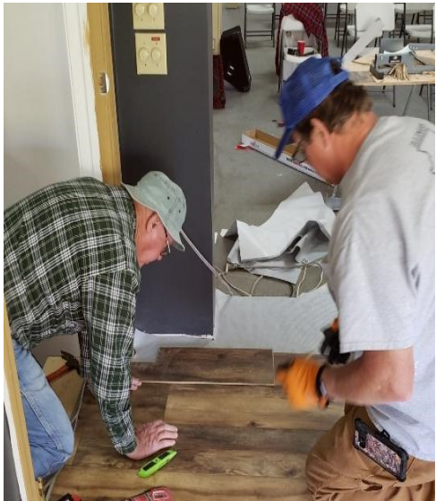
April — Lake Sallateeska Camp—laid laminate flooring on chapel stage and much more.
